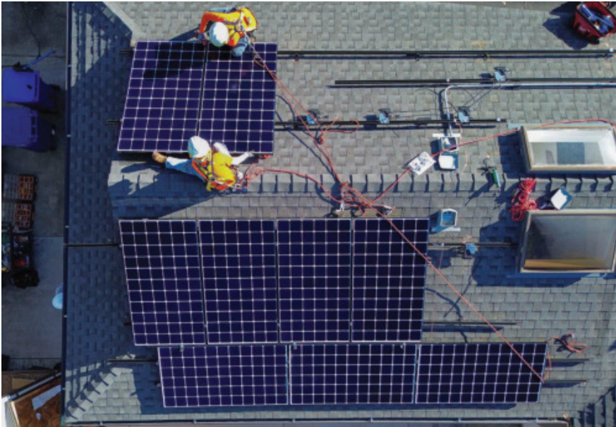
Workers install solar panels on the roof of a California home in December
